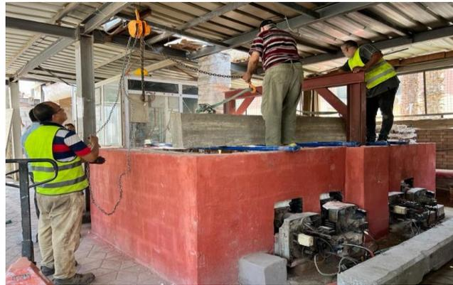
**Fig. 2:** Placing Beams in the oven
