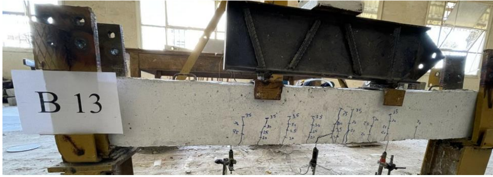
Figure 3.7: Failure mode and crack Pattern of Group 1-Conventional concrete beam reinforced with GFRP bars with different development lengths
