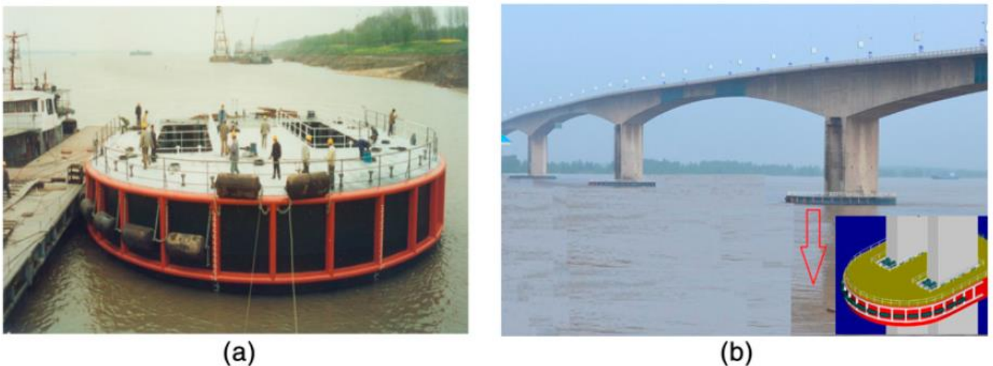
Fig. 1. (a) Floating framed steel fender system (reprinted from Sun 2007, with permission); (b) Huangshi Bridge (image by Sun Zhen)
