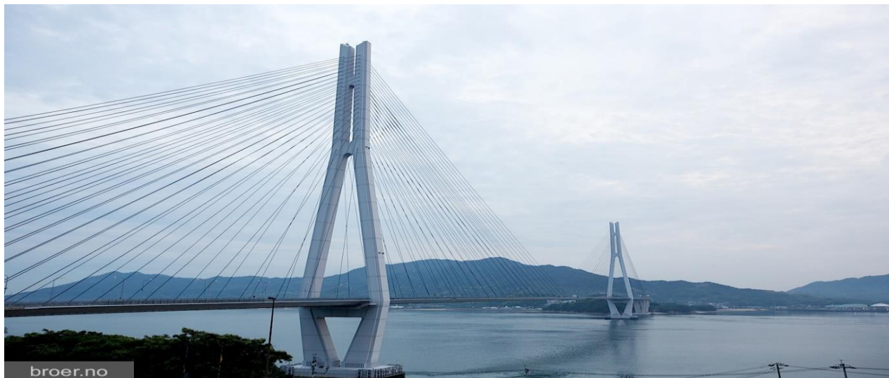
Fig. 2. Tatara Cable-Stayed Bridge
