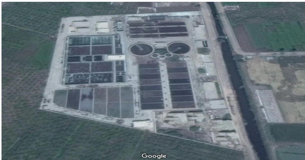
Fig. 1. Kafr El - Shahawi Khater WWTP
