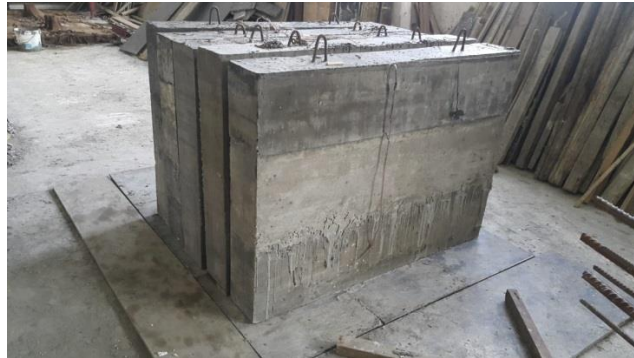
Figure 6 - Removing of formwork After 10 Days from casting
