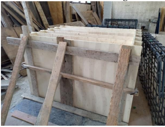
Figure 5 - Preparation of formwork
