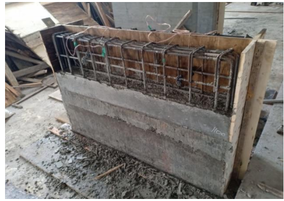
Figure 5 - Preparation of formwork
