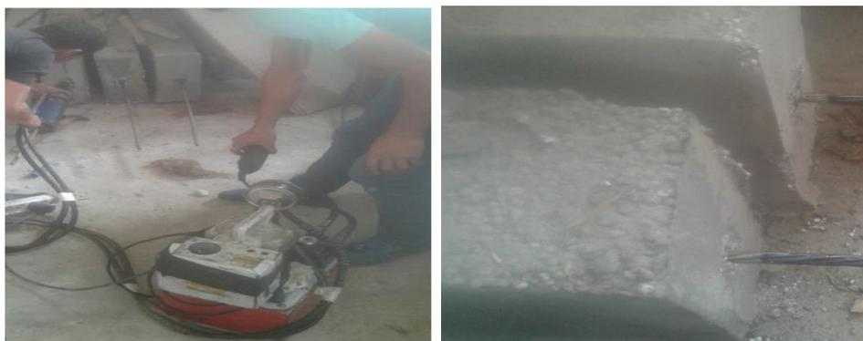
Fig 4: Application of Prestressing Force and Elongation After Tensioning the Tendon.
