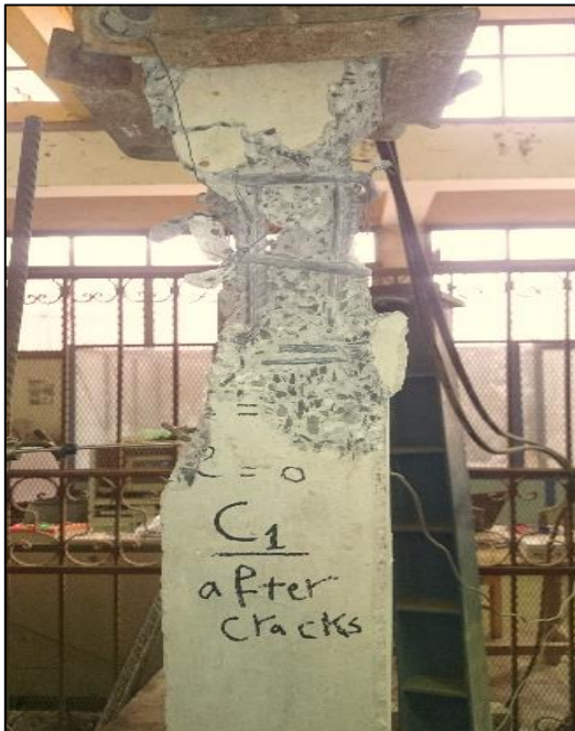
Fig. 7. Failure mode of Specimen C1
