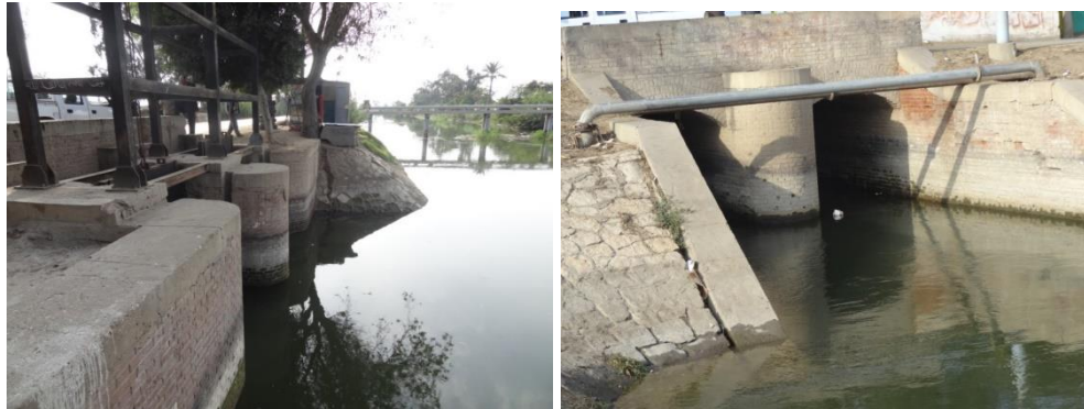
(a) upstream view
