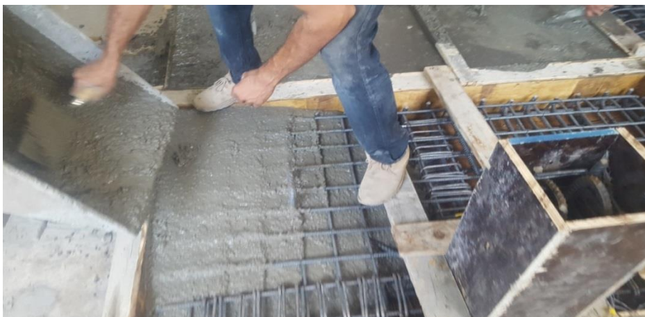
Fig.4: casting of specimen
