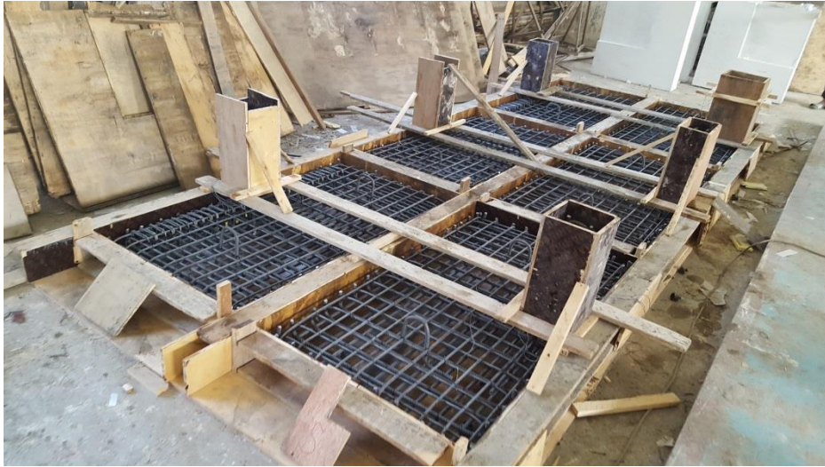
Fig.2: formwork and steel rebar
