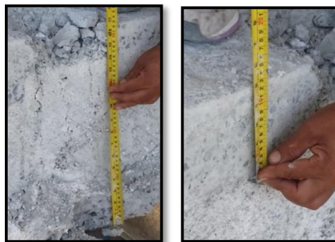
Fig.21. measuring of thickness of the rib and top slab
