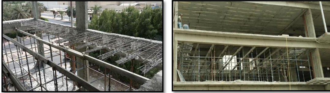
Fig.22. reinforced concrete slabs after cutting
