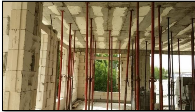
Fig. 18. Supporting the adjacent concrete slabs
