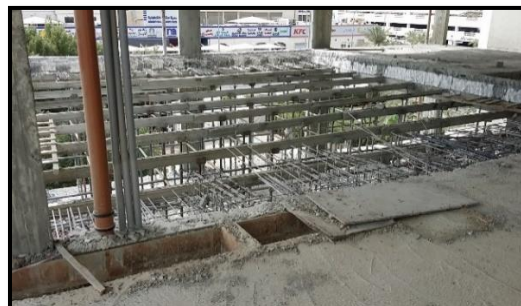
Fig.20. Reinforced concrete slabs after cutting
