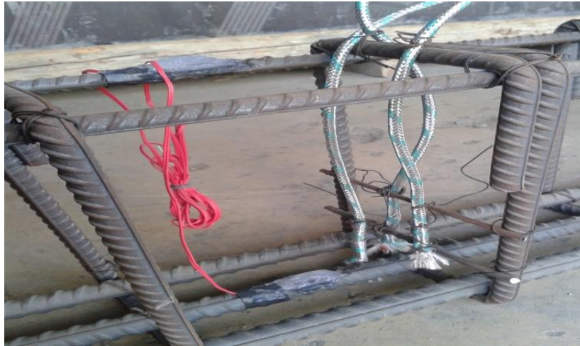
Fig. 2 Location of thermocouples at beams midspan
