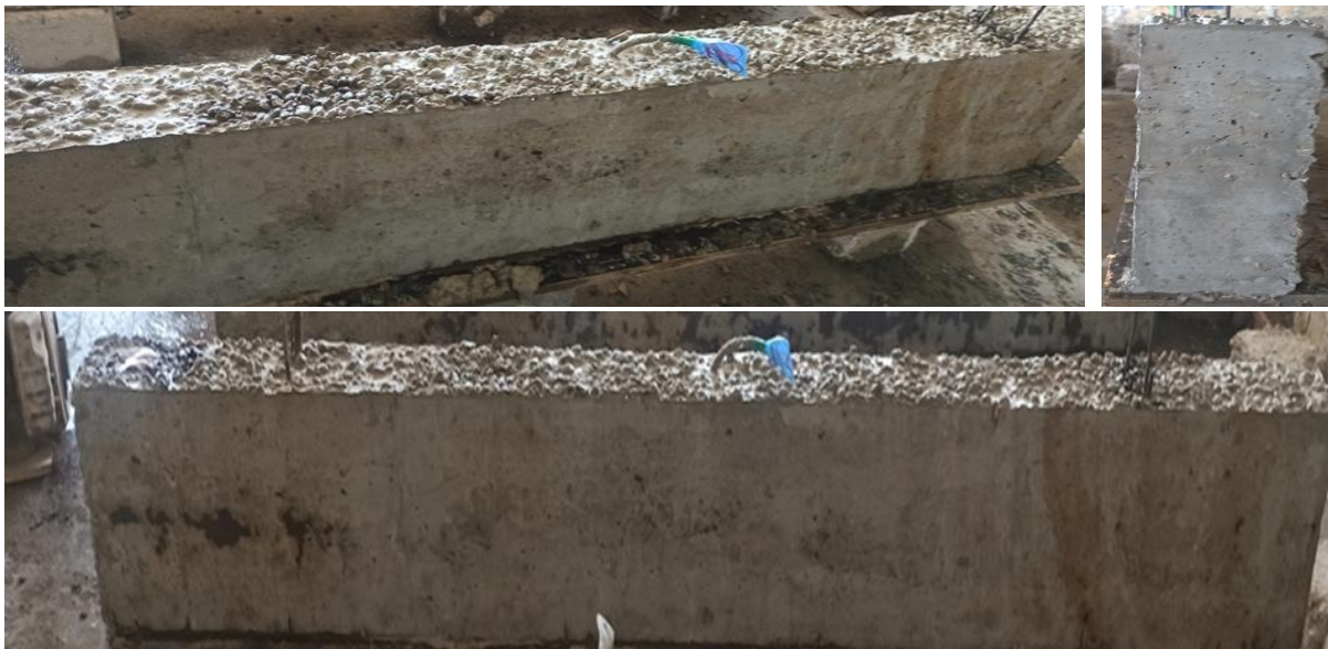
Fig. 9: The surface finish of RC beams casted with SCC
