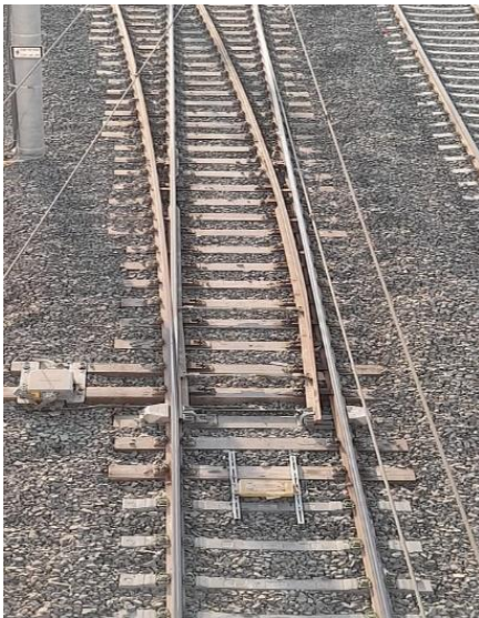
Figure (1-a). a switch panel
