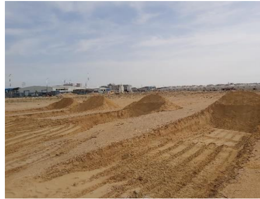
b – Digging and measuring experimental sections
