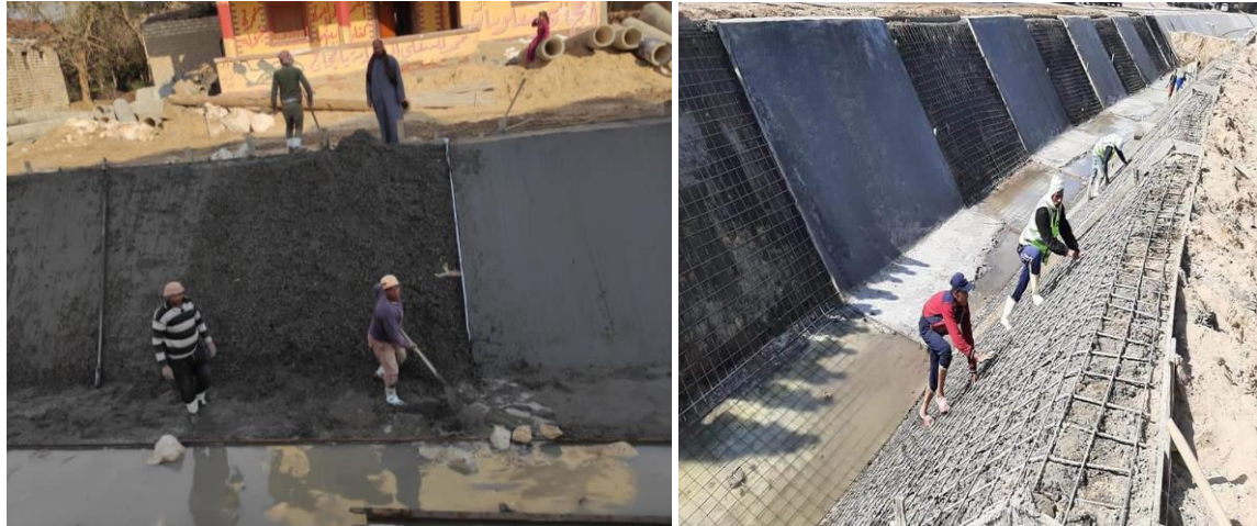
Fig. 2: Cast in place Concrete lining.
