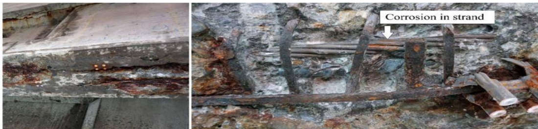
Figure (1). corrosion of the prestressing steel [1]
