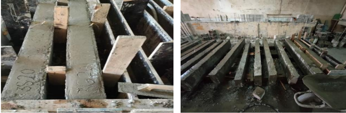
Fig. 3: Casting and curing
