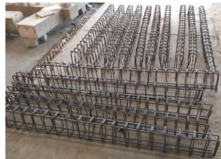
Fig. 2: Reinforcement for beam
