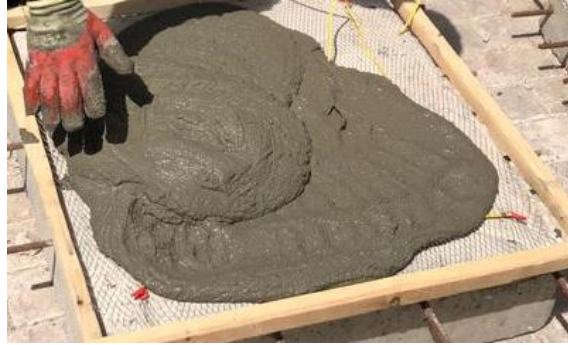
Fig. 1. protective cement paste containing ungalvanized steel mesh
