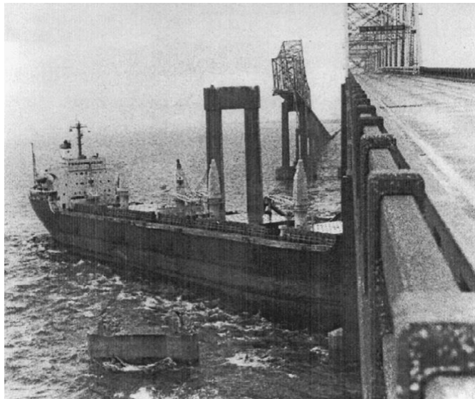
Fig. 1. The 1980 collapse of the Sunshine Skyway Bridge
