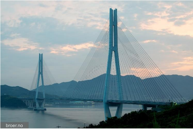
Fig. 2. Tataru Cable Stayed Bridge
