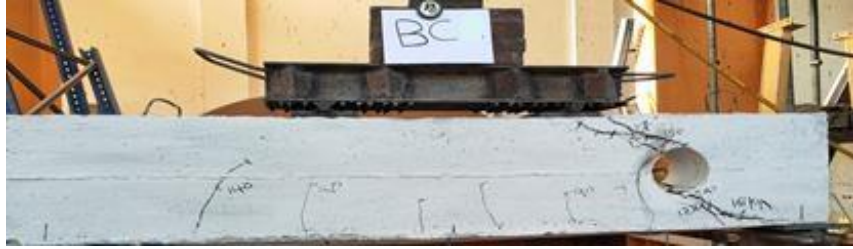
Fig. (3).Cracking Pattern for Beam (BC).
