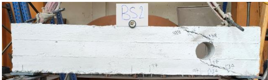
Fig. (5).Cracking Pattern for Beam (BS2).
