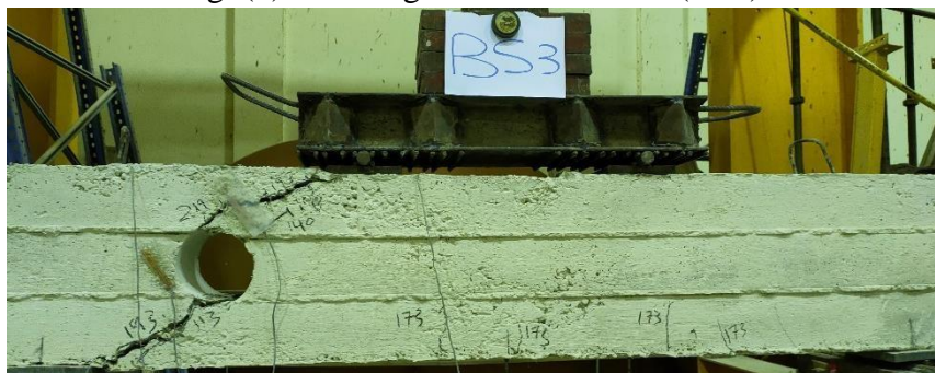
Fig. (6).Cracking Pattern for Beam (BS3).
