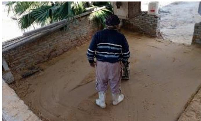
(b) sand layers compaction
