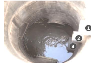
Figure (5-c) all plugs are open (pre-harvesting)
