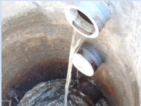
Figure (5-a) First plug is open while the second and third closed (planting stage)
