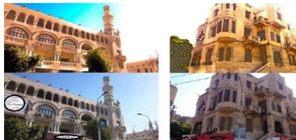
Figure (10) distortions during buildings usage - Façade's color changes
