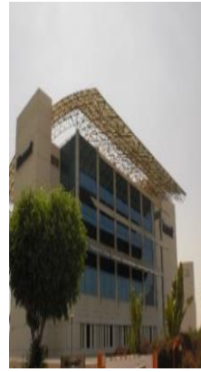
Figure (7) large external shading in the Microsoft building in Smart Village, Egypt. Source: (Author)
