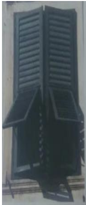
Figure (5) wood blinds of windows. Source: (Z, Salah)
