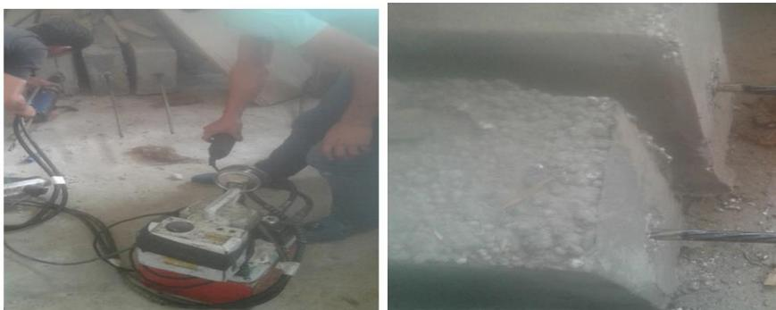
Fig. 5: Application of Prestressing Force and Elongation After Tensioning the Tendon
