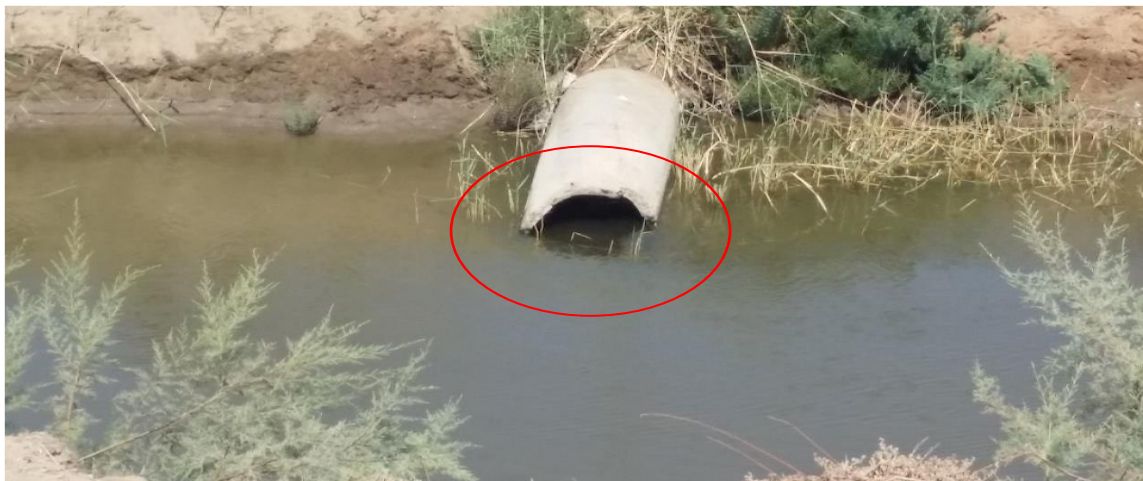
Figure 5: Submerged pipe tail escape at a secondary drain
