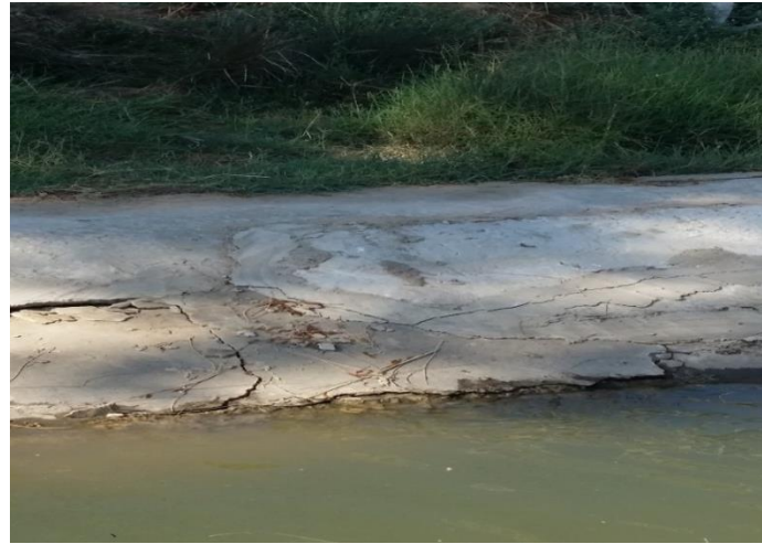
Figure 12: Sample of collapsed panels
