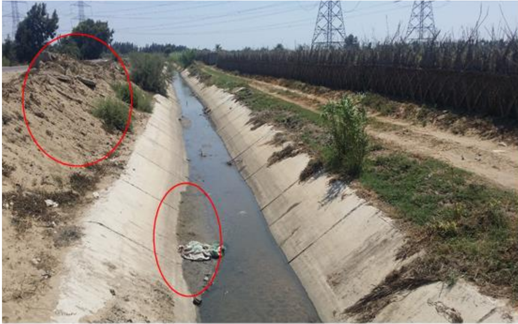
Figure 8: Sediment depositions at lined mesqa
