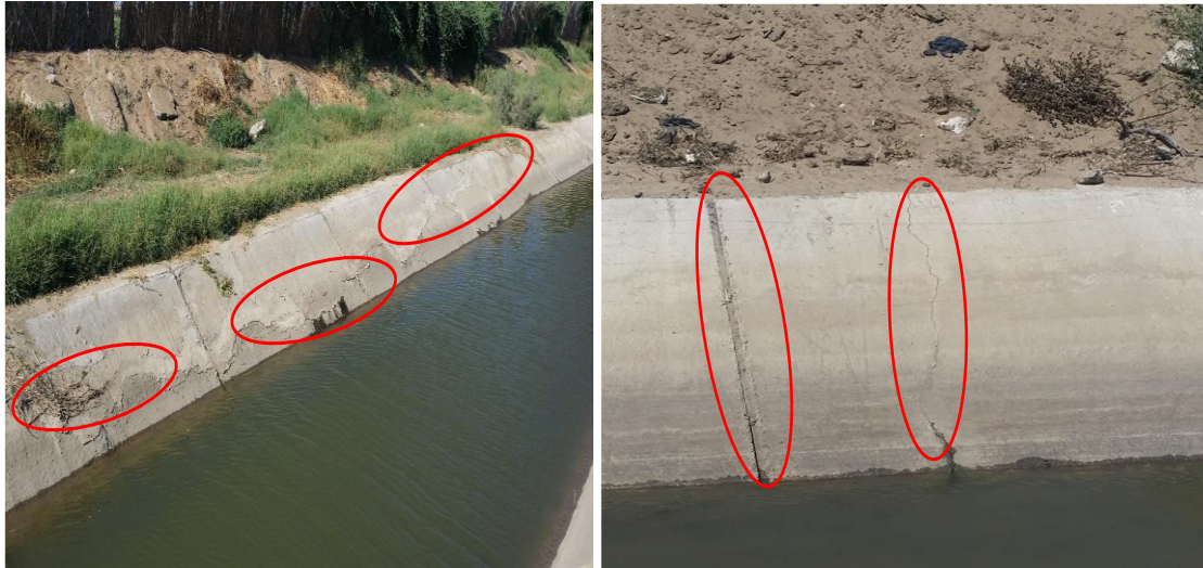
Figure 6: Damages to the concrete lining
