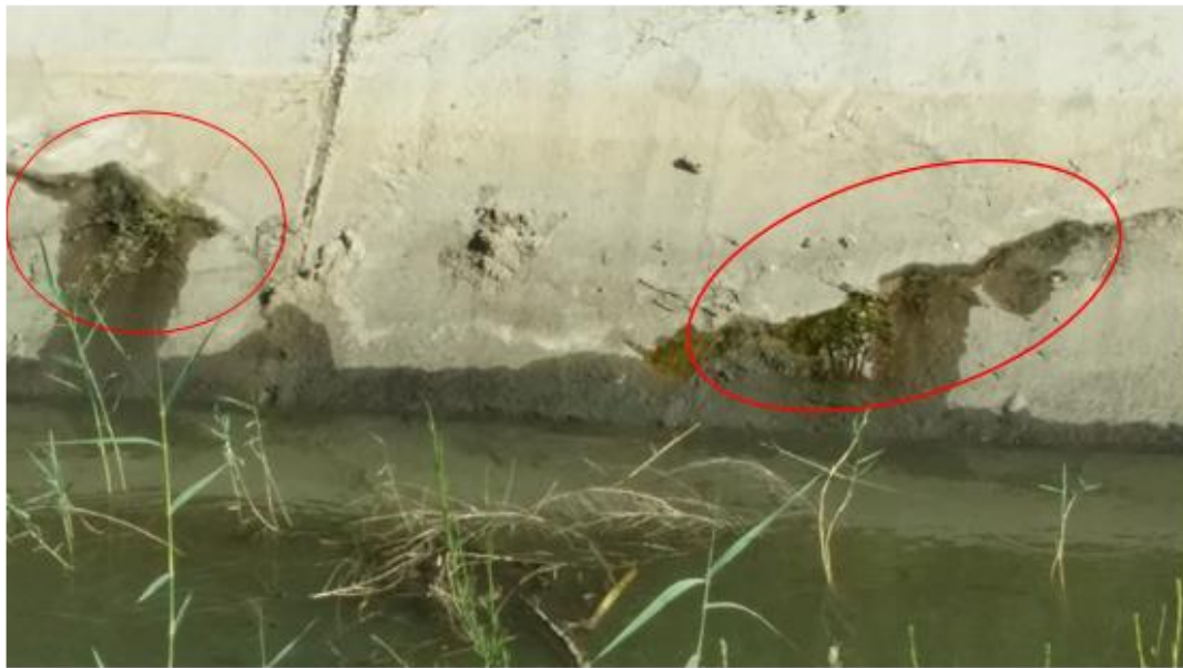
Figure 9: Seepage through the concrete lining
