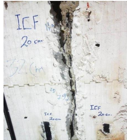
Identical cracks in EPS sheet block and R.C
