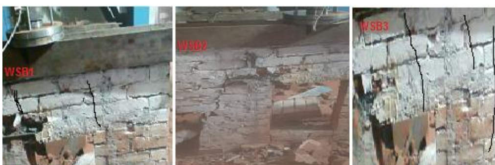
Fig. 8: Failure mode for walls strengthened with steel bars
