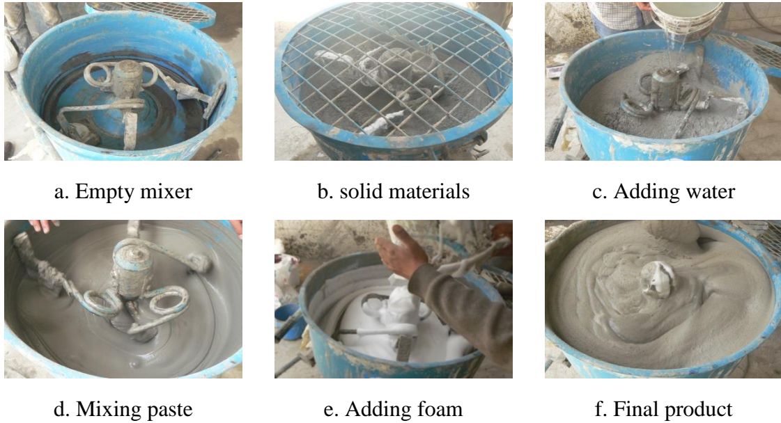
Fig. 3: Foamed concrete manufacturing process
