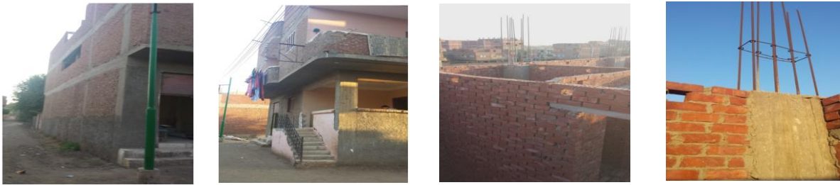
Fig.(3) Typical Non-engineered Concrete Frame with Infill Wall Building Chosen for Analysis
