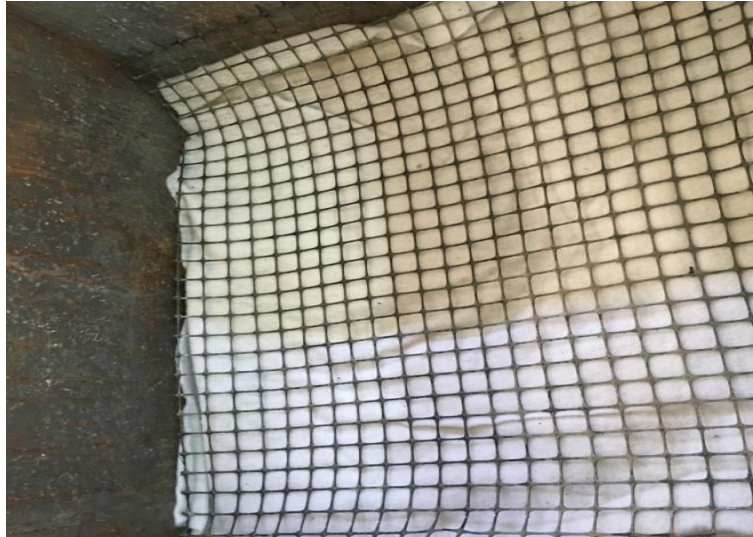
Fig.3. Geo-textile + Geo-grid sheets above subgrade
