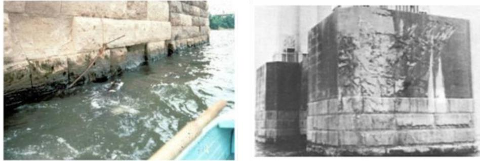
*FIGURE1. Deteriorated Masonry due to Impact*
