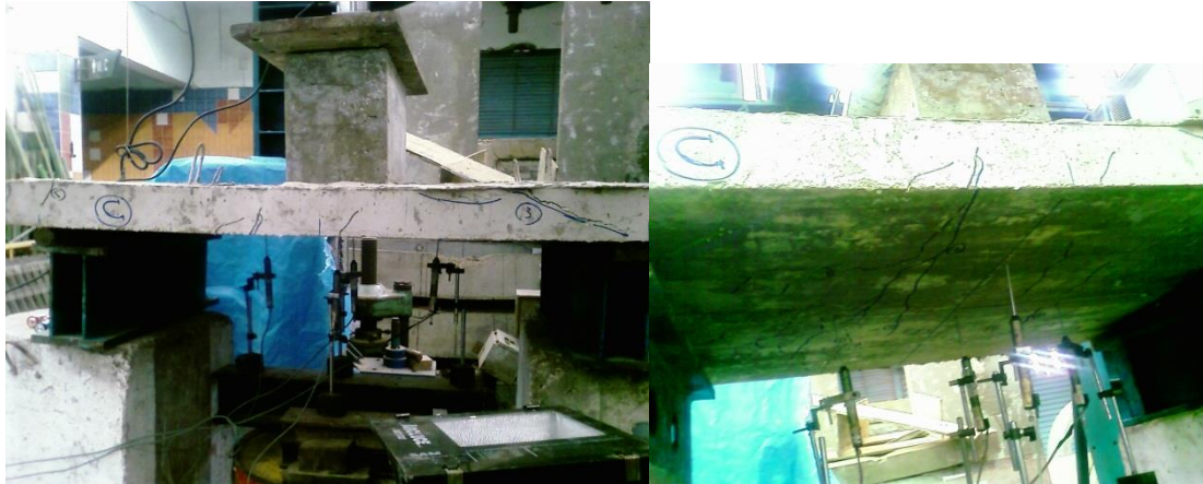
Fig. (10): Shear failure occurs accompanied with minor flexure cracks.
