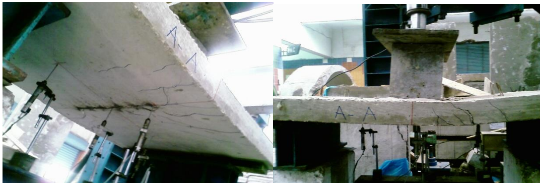
Fig. (7): Flexure failure at start of loading, at last shear failure occurs
