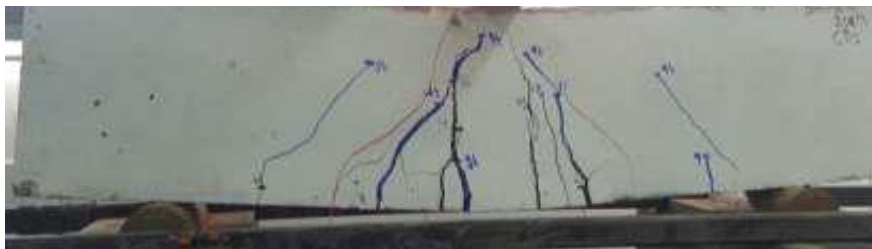
Fig. 4: Cracking pattern of control beam B1
