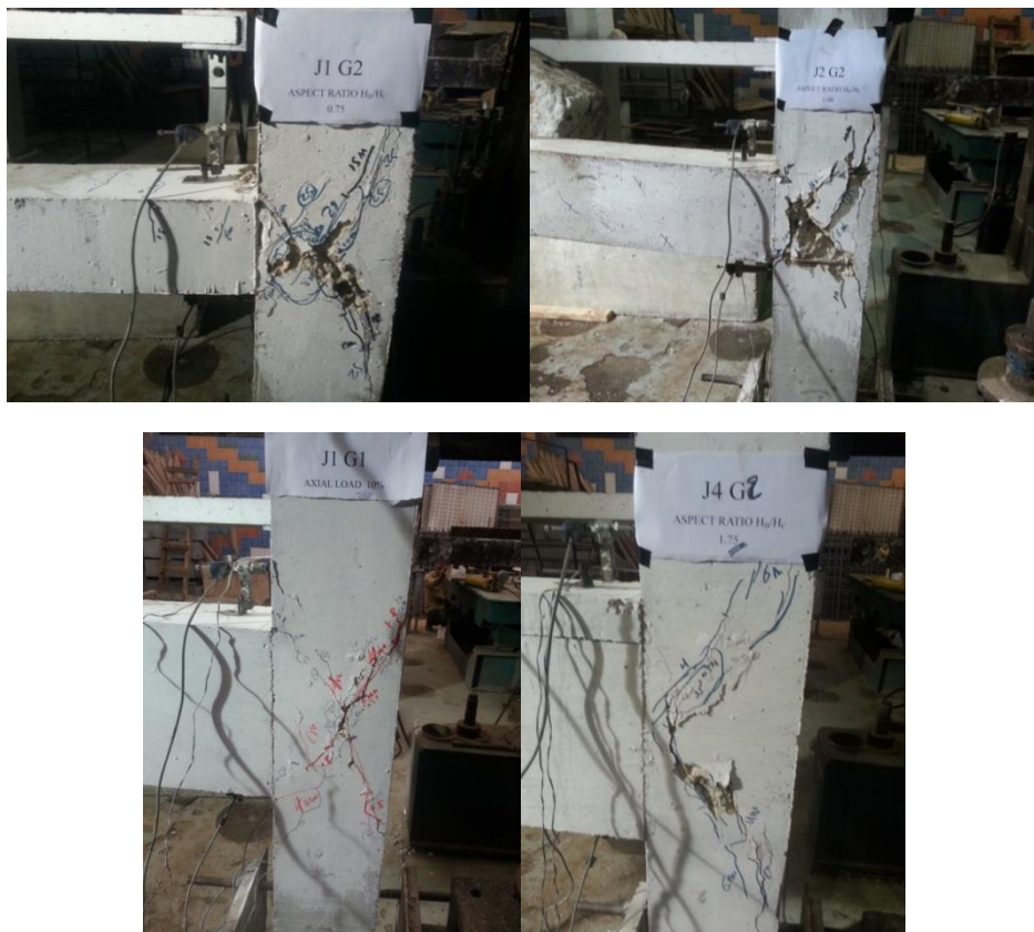
Figure 5: Crack pattern of all Specimens
