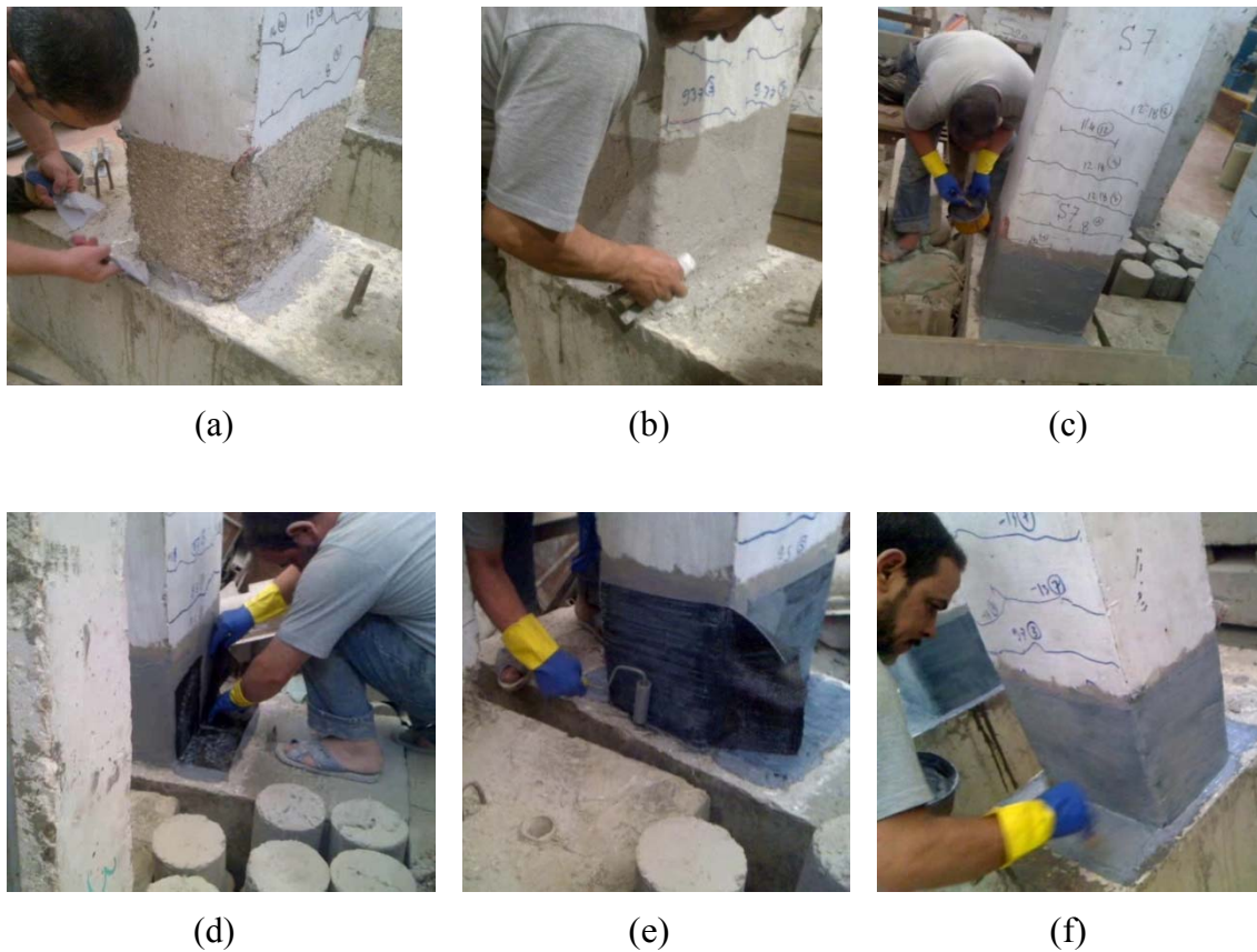
Fig. 4: Repair process, a) Application of Sikadure31CF, b) Rounded corners, c) Application of Skiadur330 d) Application of longitudinal Skiawrap230C e) Wrapping of transverse Skiawrap230C, f) Adding extra layer of Skiadur330
