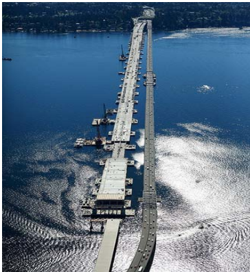
Photo (1) SR-520 floating bridge placed.
