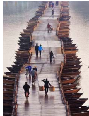
Photo (2) Congjiang floating bridge placed.
