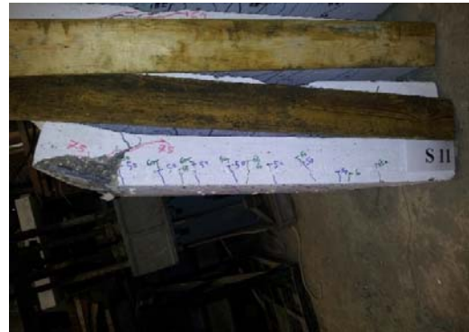
Figure 13: Shear cracks of specimen S11
